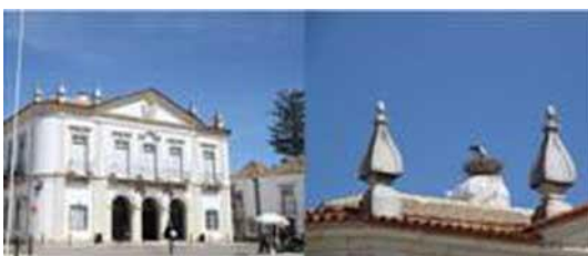
Figure 16. City Hall (site 10) (João Fonseca, March 2012)
