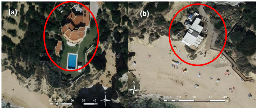
Figure 6.1 – Examples of structures with a medium and high risk present on study area: (a) Building; (b) Restaurant
