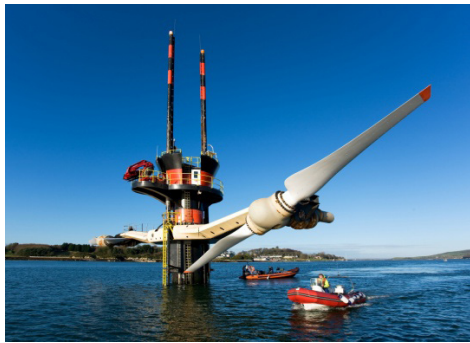
(A) SeaGen, Marine Current Turbines
