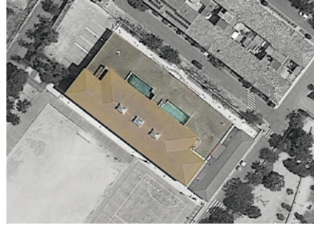
Figure 16. Volumetric classification. School S026. Building: 1. Type: compact. Sub-type: with courtyards.
