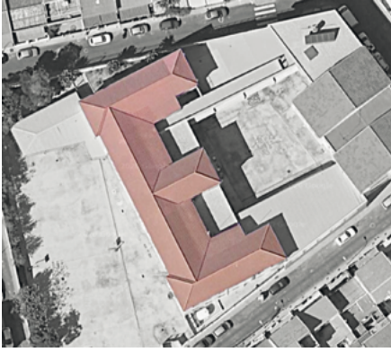
Figure 26. Volumetric classification. School S058. Building: 1. Type: intersection. Subtype: E-shape.
