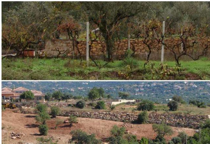
Figure 1: Upper: terrace with a dry stone support wall partially replaced by a masonry wall in the Cernache of Bonjardim area; Bottom: terrace with a recent wall, built with regular stones of exaggerated dimensions for this context, Algarvian Barrocal (authors)
