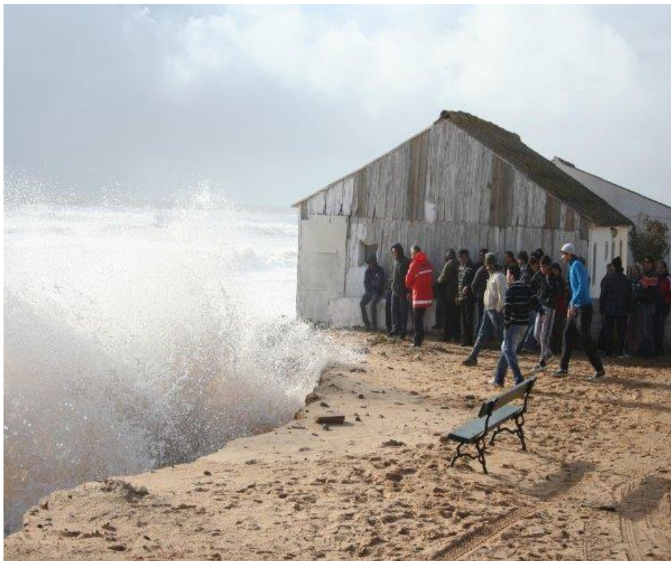
Figure 2.1 – Storm at Faro Beach that led to loss of houses in 2010 (the house shown here is the same as in Figure 2.2). Source: http://adefesadefaro.blogspot.pt/2011/02/ilha-de-faro-sob-risco-iminente.html (used with permission).
