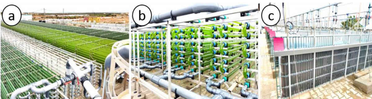
Figure 1.7: Closed systems for the production of microalgae at the facilities of Necton S.A., Olhão. Tubular PBRs (a,b) and vertical panels (c) known as "flat pannels" or "greenwalls" (Photos by Britta Kautzmann).
