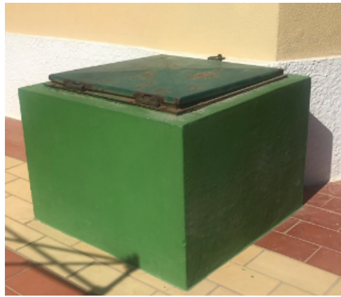
Figure 2.6 Existing RHW systems located in the Social Centre of Culatra Island.
