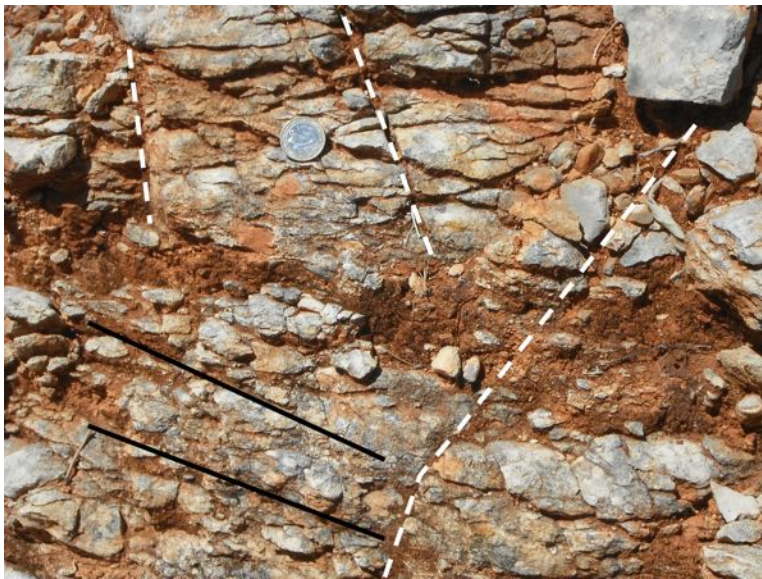
Figure 7.1. Alteration in the limestone of the Escarpão Formation. The fractures represented with white dashed lines and the layer planes represented with black lines make it easy for water to penetrate. Note that the layer planes are almost completely obliterated due to the alteration. The alteration results in limestone fragments and red clay ( terra rossa ). The two forms of weathering – chemical (dissolution) and physical (fracture) – contributed to the alteration of this outcrop.
