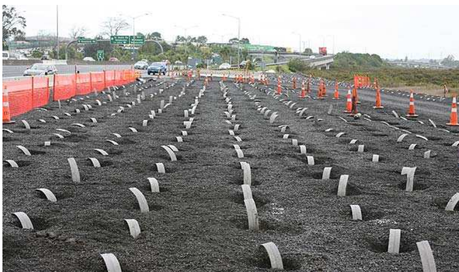
Fig.20 – Corte do dreno aplicado a cota apropriada (retirado de http://www.stuff.co.nz/auckland/local-news/western-leader/9522556/Wick-thinking-underpins-motorway-sea-water-drainage-process , em Novembro de 2014)
