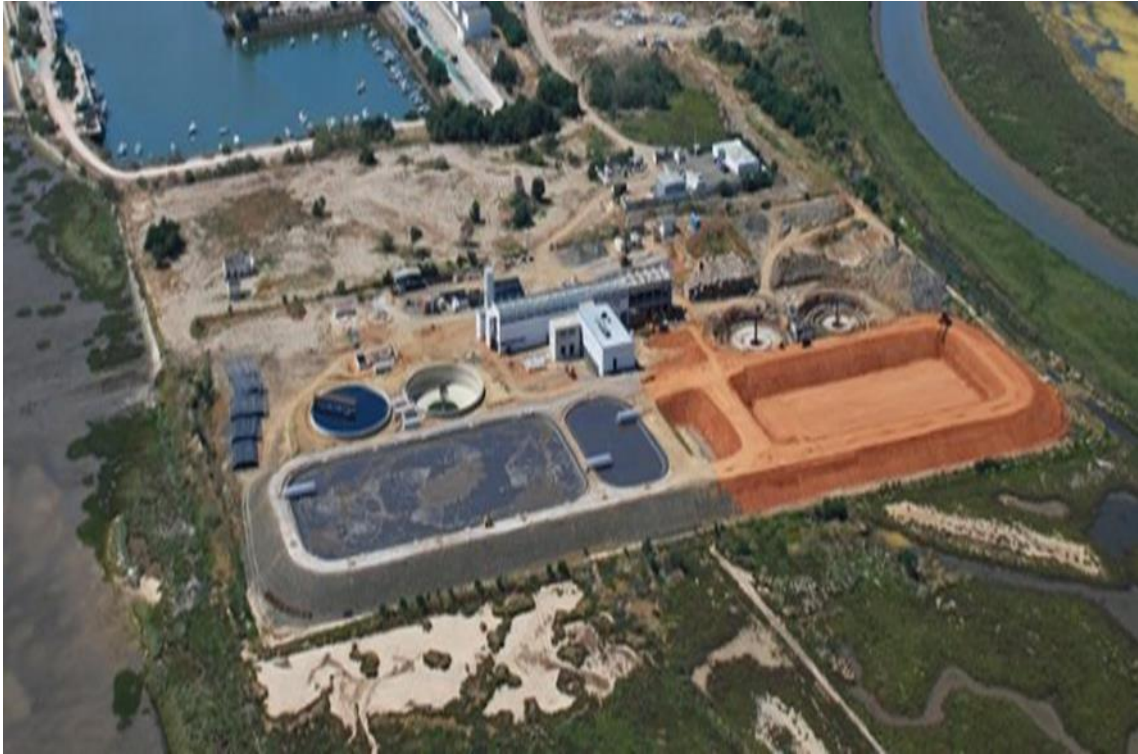
Figure I.10. The Area view of Vila Real de St. António WWTP (Águas do Algarve, 2025)
