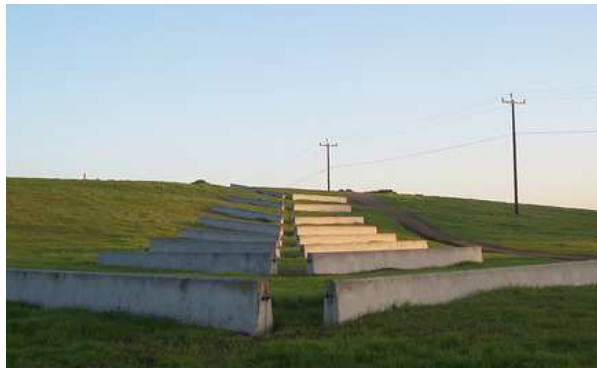
Figura 28 – Blocos de betão ( http://farm1.static.flickr.com )
