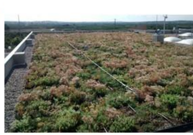
Greenroof in Benaguasil (Spain)
