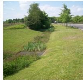
Filter strip leading to wet swale in Scotland
