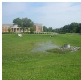
Infiltration basin in Cincinnati (USA)
