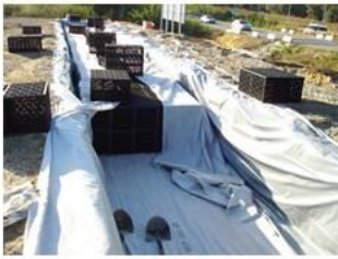
Construction of a geocellular system in Oleiros (Spain)
