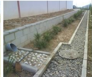
Filter drain in Crevillent (Spain)
