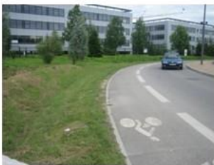
Vegetated swale in Lyon (France)
