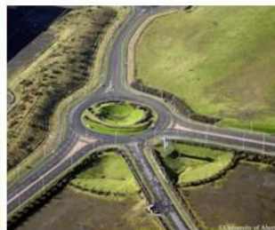
Detention basin in Dunfermline East Expansion (Scotland)
