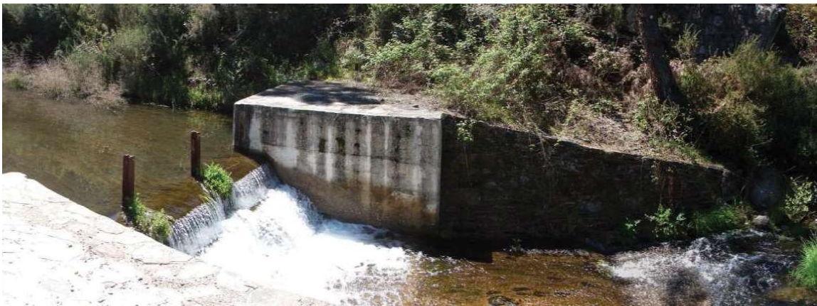
Figure 7. One of the weirs in Cerdeira creek (authors).
