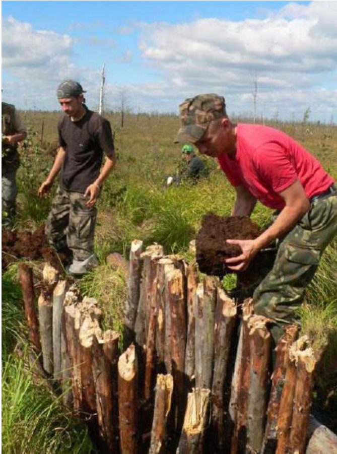
Figure A28. Dam construction process
