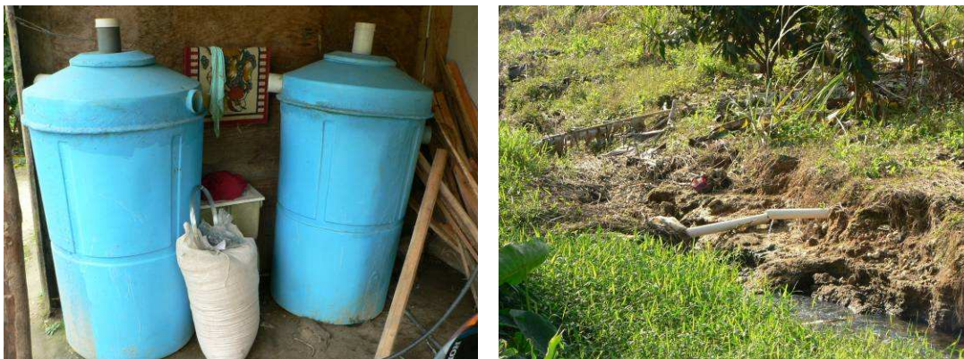
Fig. 26. Left, a cesspit kit ready to put in place, has been provided to a household through the project Microbacias II. Right, domestic wastewater entering the river through pipelines continues to have negative impacts on water quality in Brilhante.
