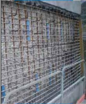
Mapeshield I applied to a viaduct pile under repair
