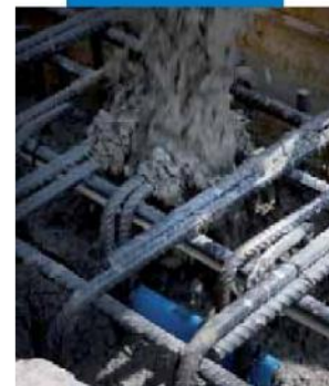
Pouring concrete for a structure protected with Mapeshield I
