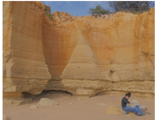
Figure 11: An open carved sinkhole with cemented walls at the western end of Maria Luísa beach (STOCK 2019).
