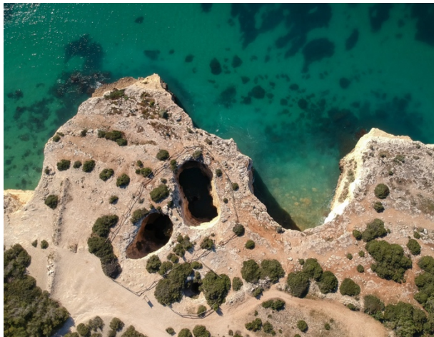
Figure 10: Two openings of a large sinkhole in the cliffs near Albandeira beach (STOCK 2019).
