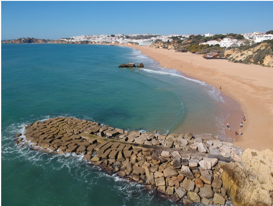
Figure 37: Groin at the eastward end of Alemães beach to prevent sediments from following the longshore drift and thus promoting accretion at the beach (STOCK, 2020).
