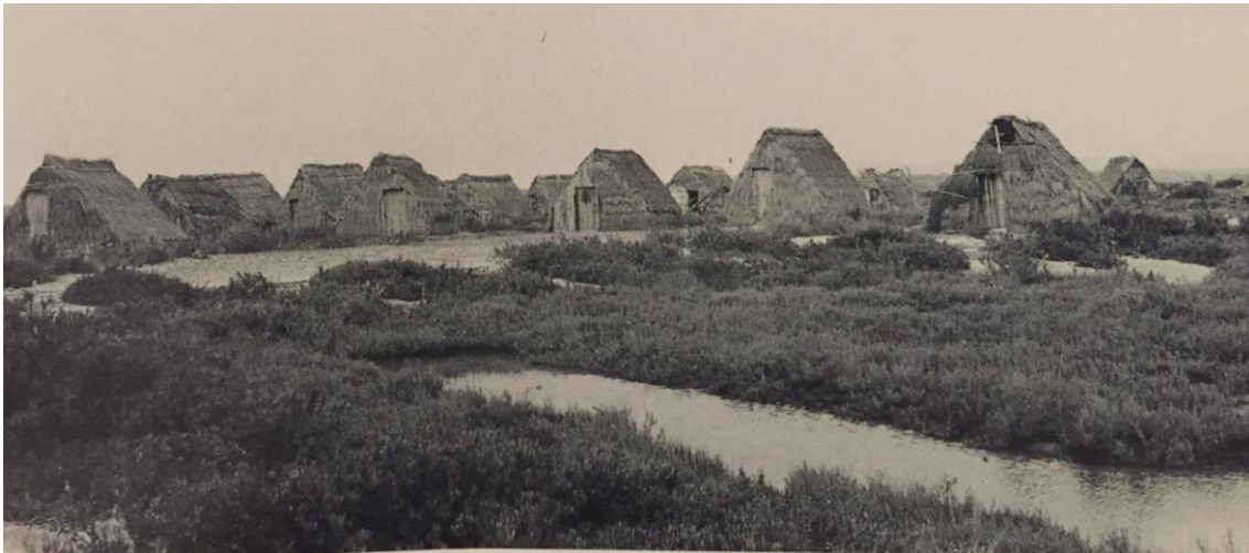
Figure 5. Former set of traditional cabins in Fornico, Faro (Source: Oliveira, Galhano and Pereira, 1994)
