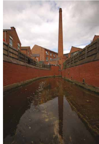
Figure 1. Canalized/culverted urban habitats, Leicester, UK.
