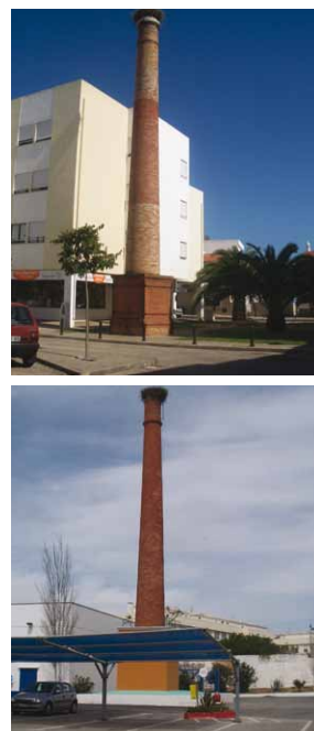
Figures 1. and 2. Examples of industrial building symbolic preservation in Algarve.
