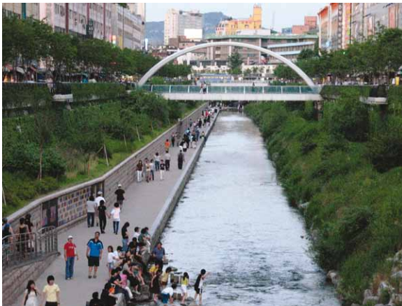
Figure 2. After dismantling of the elevated highway and structures covering the Cheonggyecheon in Seoul, Korea, the river was restored as a human-oriented, environment-friendly urban space with a waterfront and walks along the banks (Lee, 2004).
