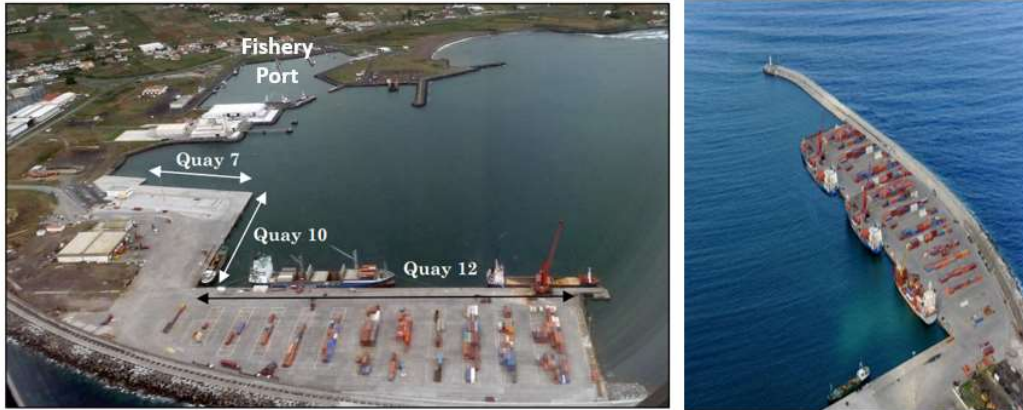
Figure 2.3- Quay wall arrangement of commercial harbour (left), and aerial view of container yard and south breakwater(right) in Praia da Vitória.
