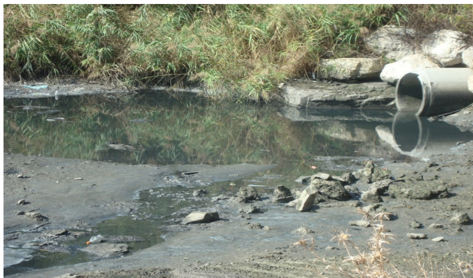
Figure 2: Sewage discharge point near Algeciras Mayorga Bridge
