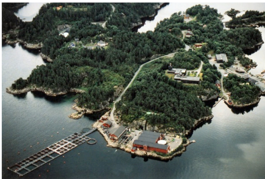
Figure 3 Picture of Institute of Marine Research, Austevoll Research station showing the facilities.
