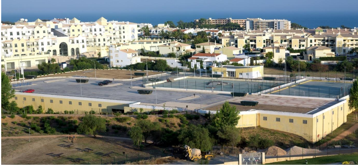
Figure 3.3. Picture taken from the outside of the Vale Faro WWTP showing the parking lot above the plant
