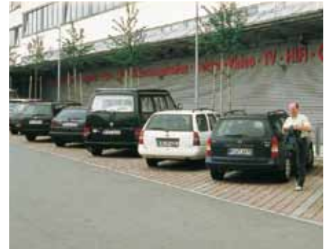
Fire brigade accessible asphalt surface.
