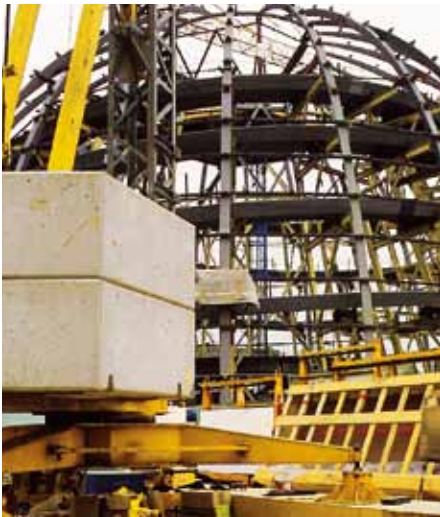
During the construction phase flat roofs are often used as storage space or place of constructions machines such as on the roof of the Reichstag in Berlin.
