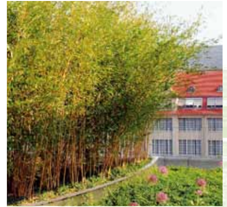
Even Bamboo can be applied on a roof but requires special safety measures.
