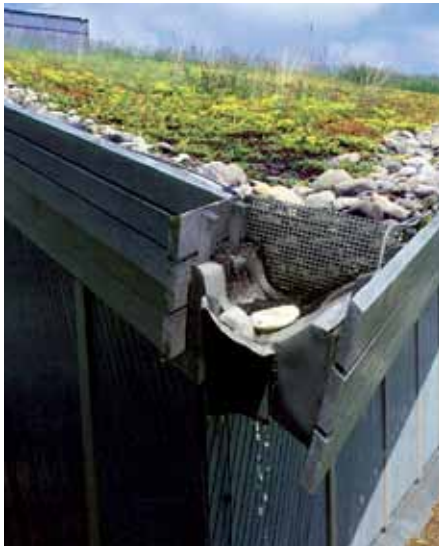
Controlled run-off in an extensive green roof
