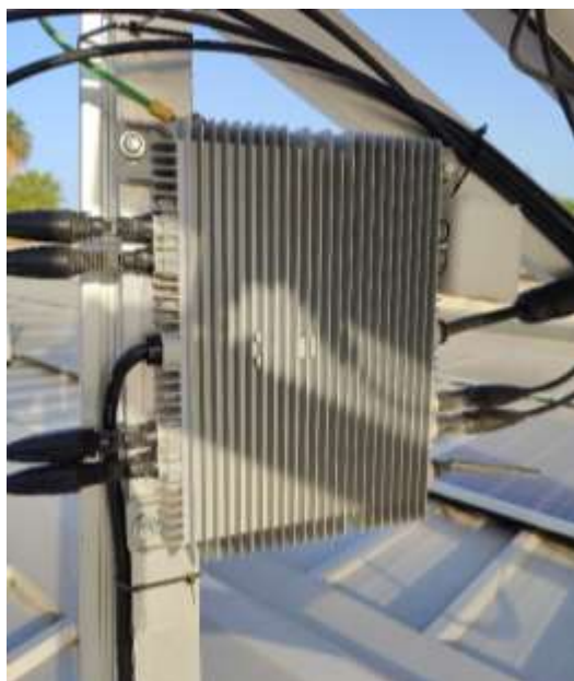
Figura 3.44 - Microinversor Deye SUN2000G3.
