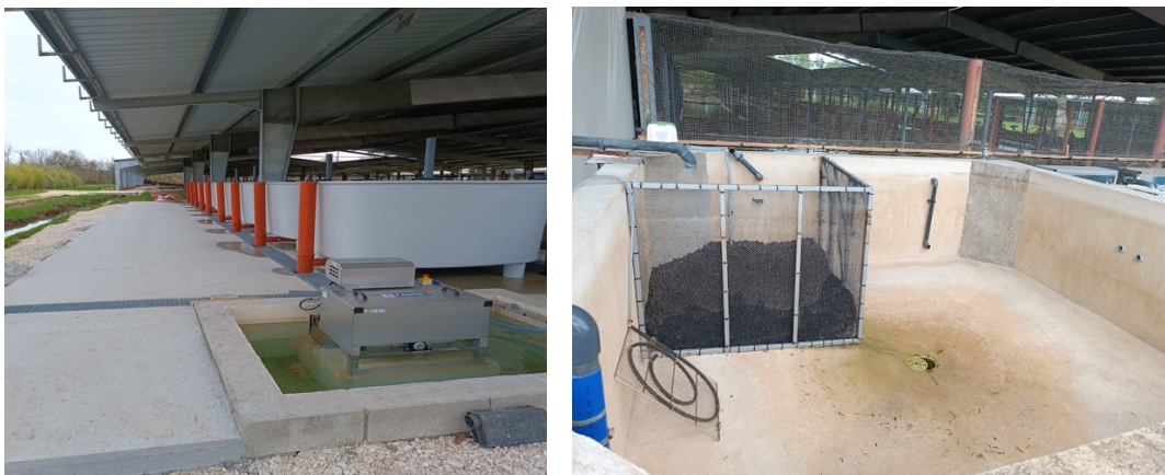
Figure 3.7: Assembled water circuit containing 9 polyethylene tanks (3.7 m 3 ) equipped with 2 reservoirs, aquatic heaters, UV, particulate, & bio media filtration
