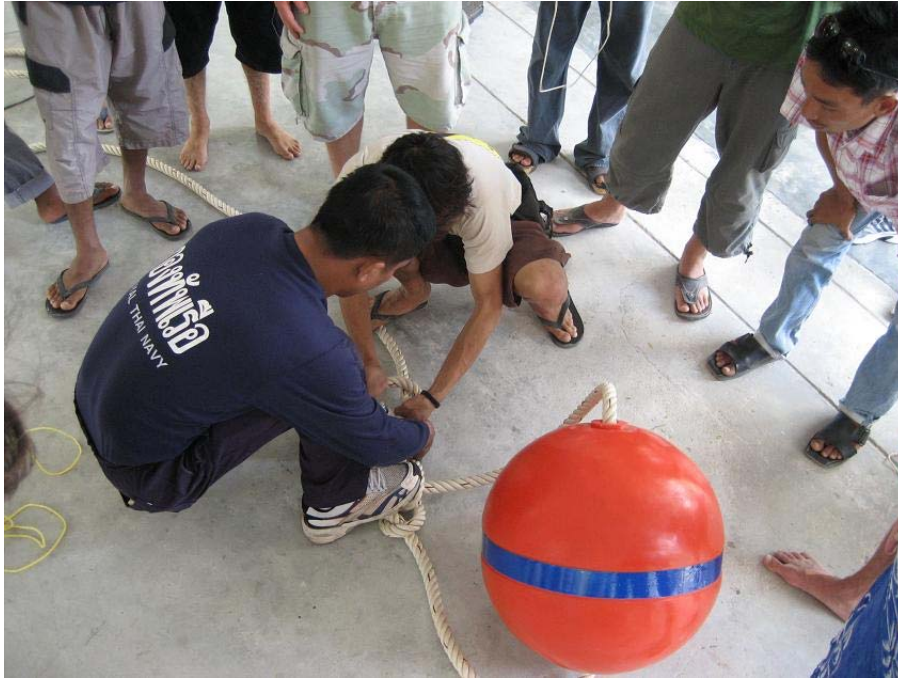
Mooring buoy assemblage to replace and install new ones on the dive sites
