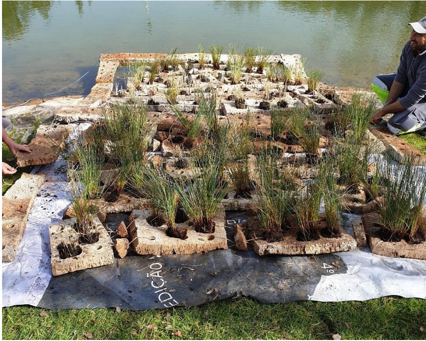
Figure 23. Putting plants into holes in cork boards (Picture taken by author on 22.02.2023)
