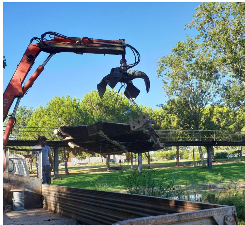
Figure 30. Island design 2 being deployed by crane (picture taken by author on 22.08.2022)
