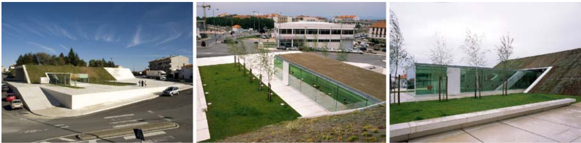
Figure 9. Mogadouro’s Bus Station (Source: http://cannatafernandes.com )
