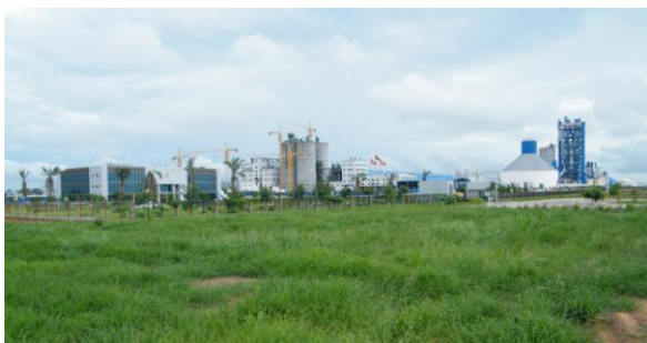
FIG 4.7 Fábrica de Cimento CIF Luanda Cement Limited
